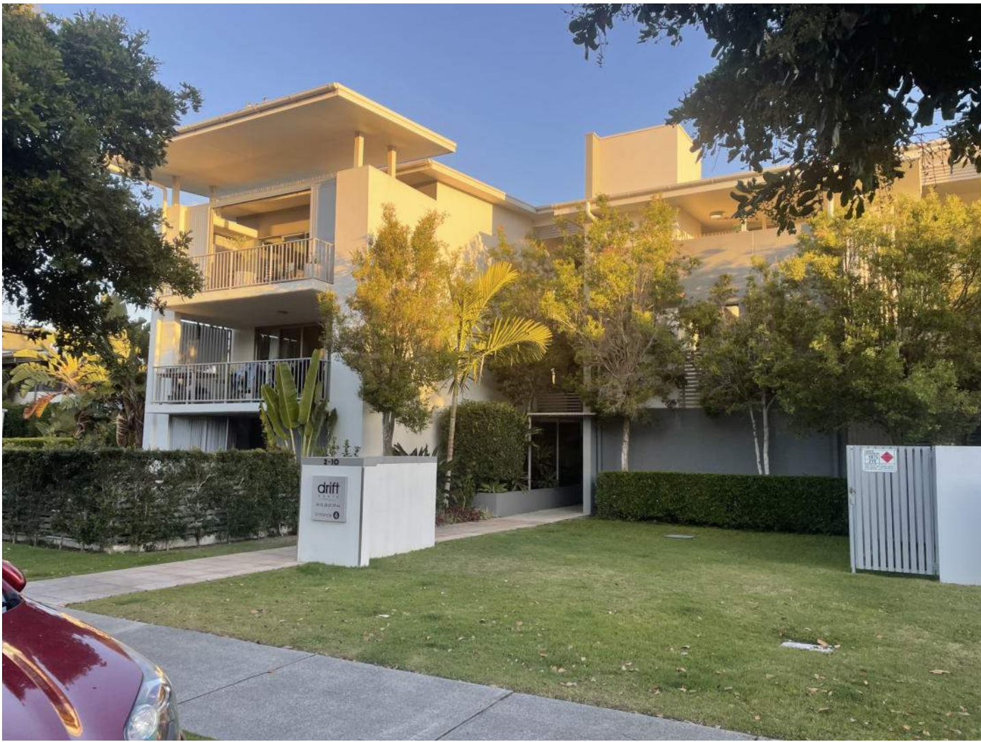
2 drift Apartments 2-10 Kamala Crescent
