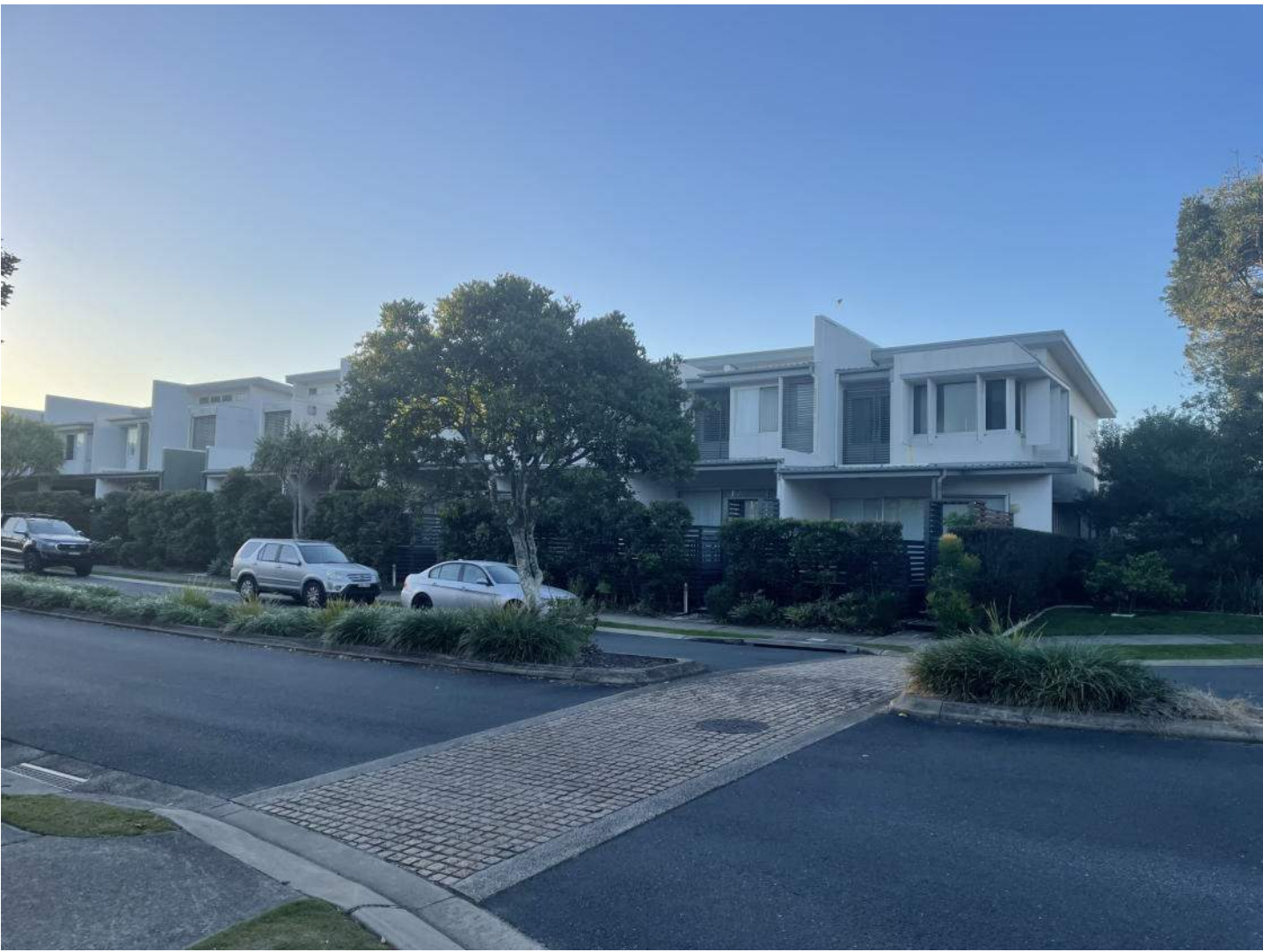
2 drift Apartments 2-10 Kamala Crescent
